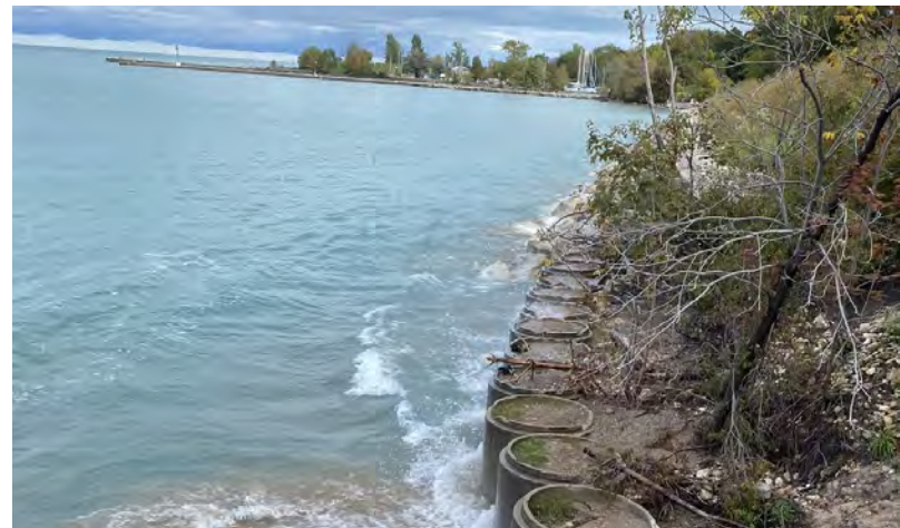
Changes in lake levels have drastically reduced the amount of beach area in Bayfield. Extensive shoreline protection projects have been completed or reinforced to protect the bluff from toe erosion.
