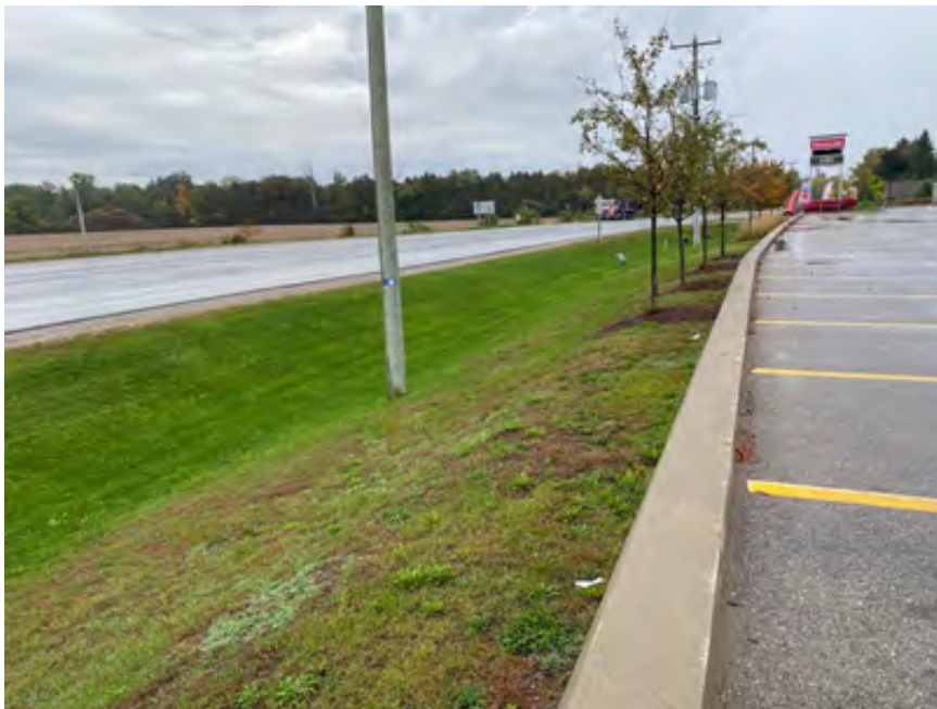
The existing ditching treatment on the west side of Hwy 21 leaves little space for an active transportation corridor.
